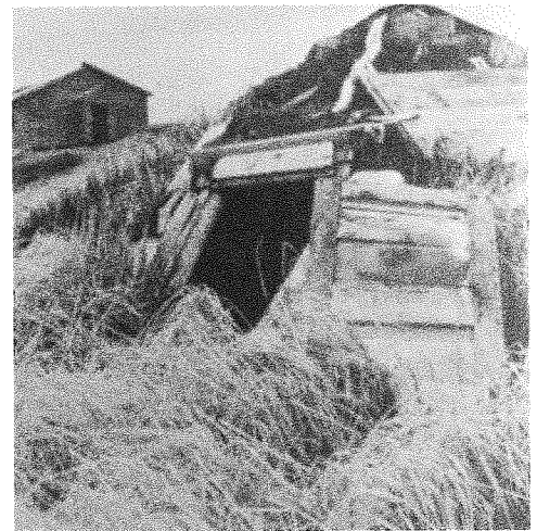
Early homes in the Aleutians were made of driftwood and sod and were partially underground. They were called "barabaras."
