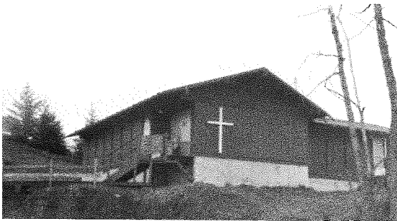
The original building in Seldovia was damaged by the 1964 earthquake and so was replaced by this building, built with earthquake relief funds in 1976.
