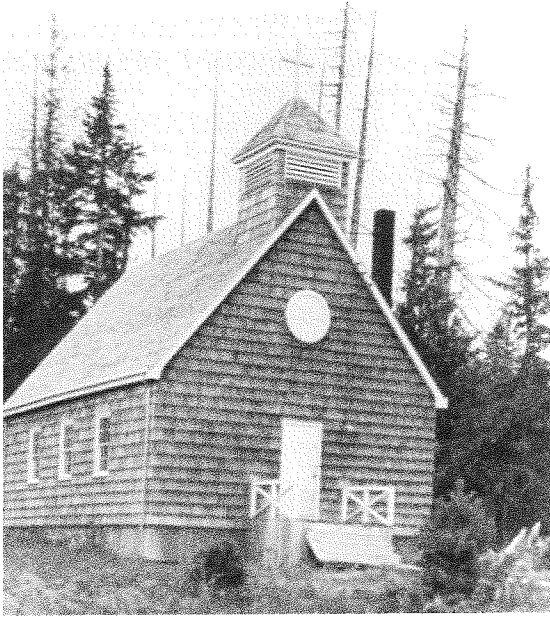
A truly neat little church building, the Clover Pass church was sold in the late 1970's.
