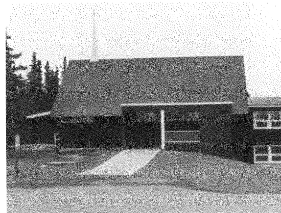
Development of the oil industry on the Kenai contributed to the growth of the Kenai church.
