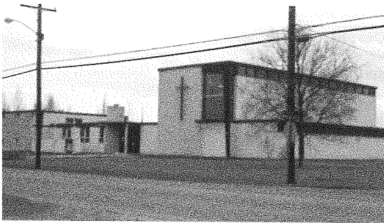
Completion of the education unit made it possible to remove the temporary building and proceed with landscaping.
