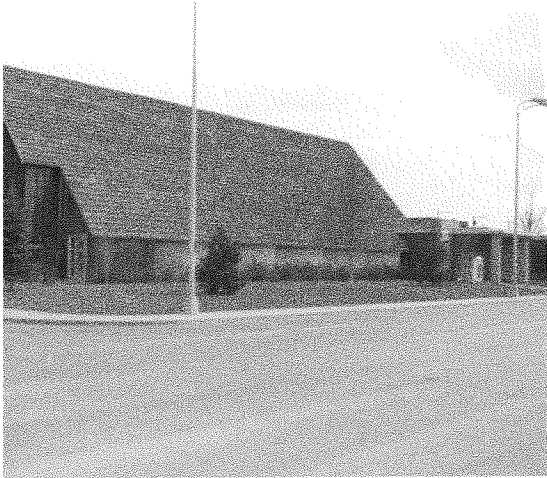
First Methodist Church, Anchorage. The education unit can be seen at far right in the picture.
